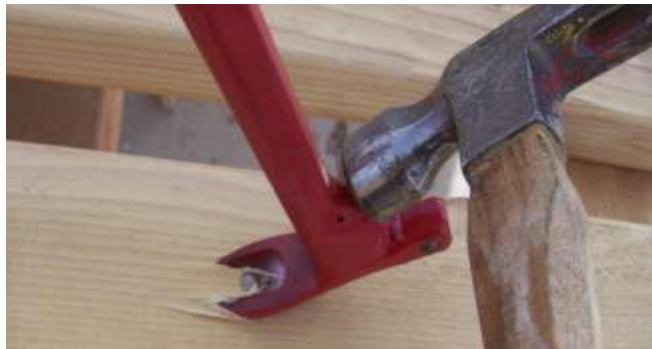
Digging out and pulling a nail
